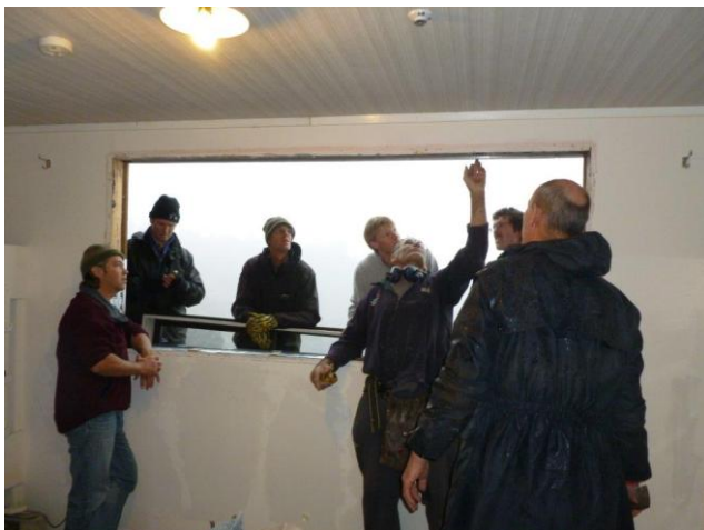
Installing the new window in the end bunk room.
